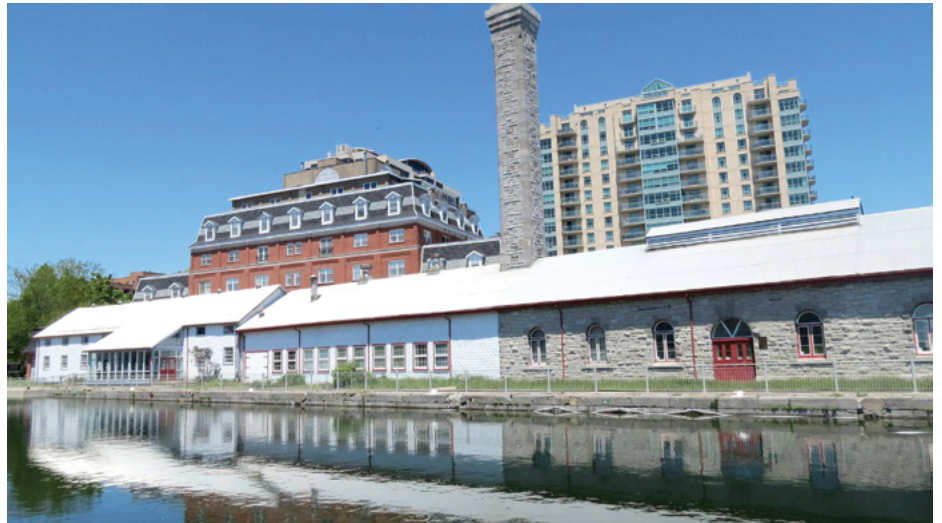
Empty drydock at the Marine Museum of the Great Lakes in Kingston which the Alexander Henry occupied for more than 40 years and will eventually be occupied by Keewatin. Photo By Pat Brennan.
