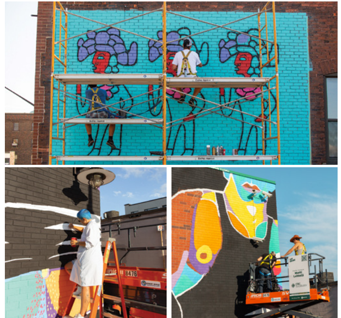
Working in progress. Photo provided by UP Here.
