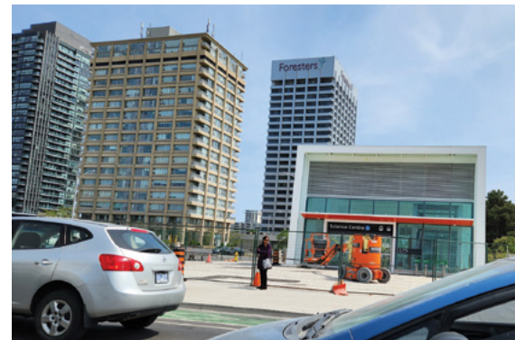
Ontario Science Centre new transit station entrance . Photo by Andy Manahan.
