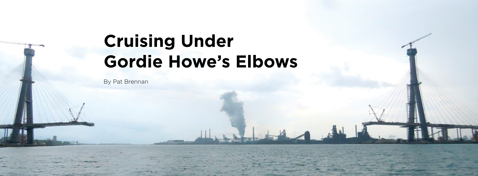
Gordie Howe International Bridge under construction . Photo by Pat Brennan.
