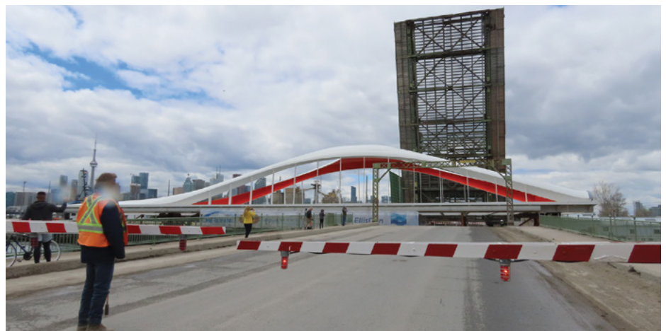
Bridge being installed connecting Cherry Street to Villiers Island.
